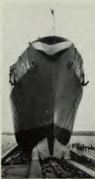
NEW AND TENDER—Polaris submarine tender, Canopus (AS 34) slides down the ways during launching.
